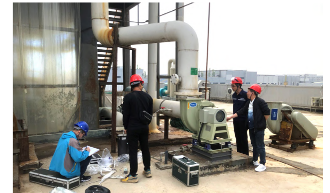
Exhaust monitoring by a third-party agency
